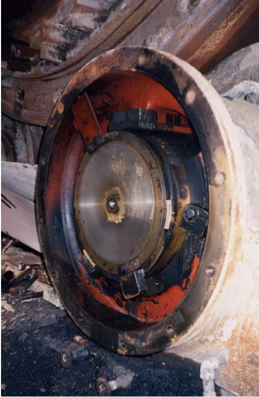
Photo #2 - Condition Survey of Kiln Trunnions
