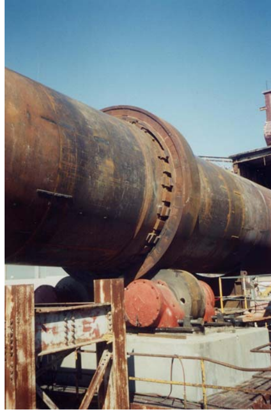
Photo #5 – Installation of New Kiln Shell Section
